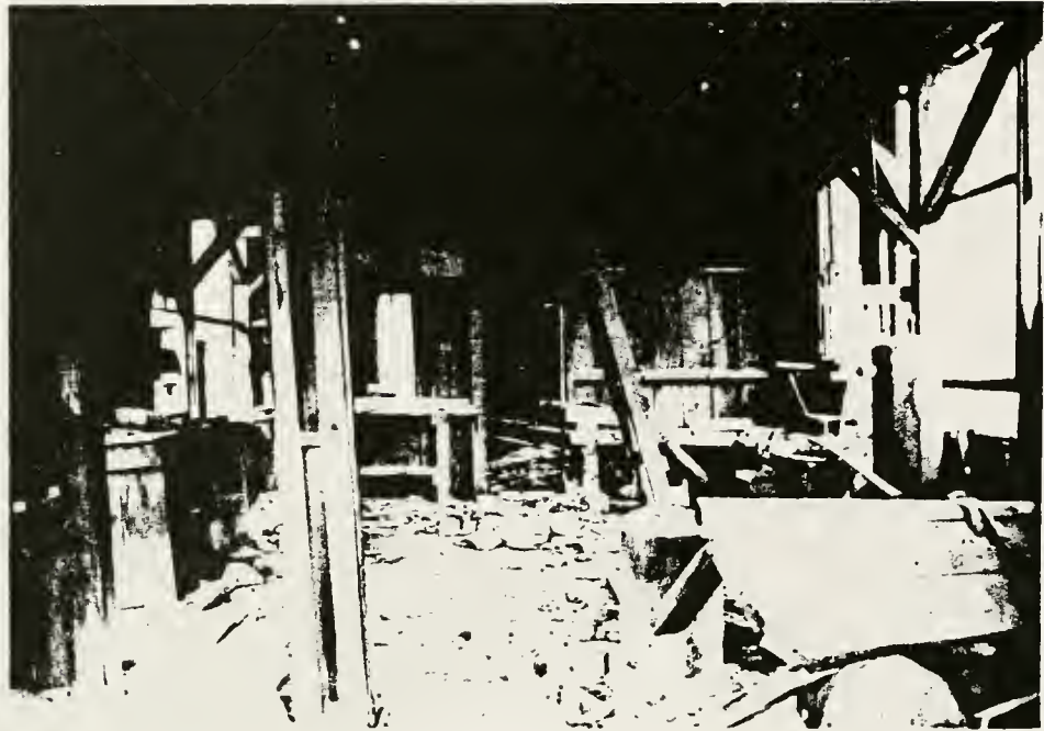
Figure 148. Interior of Assay Office (structure #58), north view.
